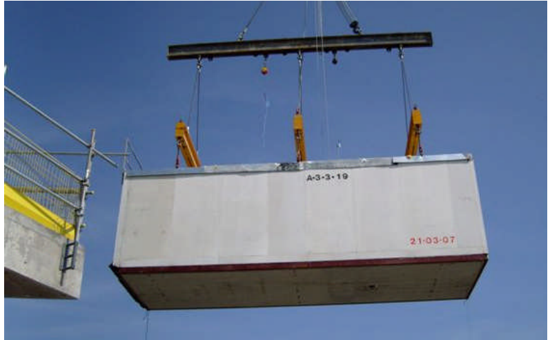
Lifting Module On Site
