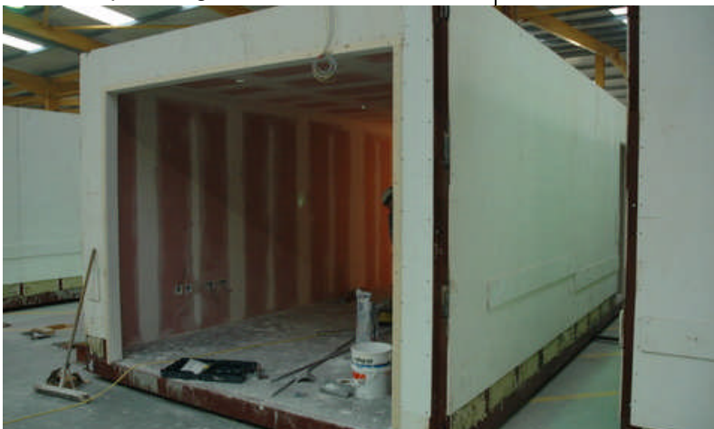
Module Construction in Factory
