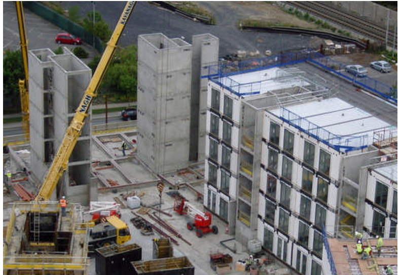
Cores and Modules under Construction at Rockbrook
